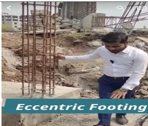
Training to the Students for Importance of Field education (how to read the Drawing, Site supervisor” by Dr W N Deulkar
