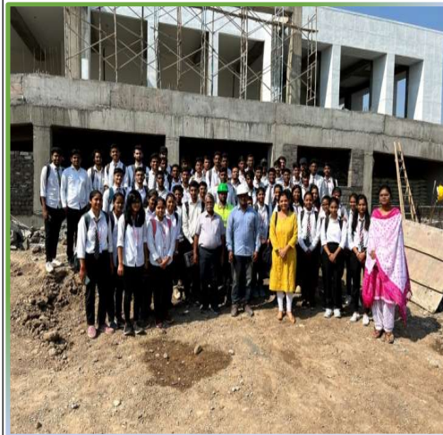
Training to the Students for Importance of Field education (how to read the Drawing, Site supervision” by Dr W N Deulkar
