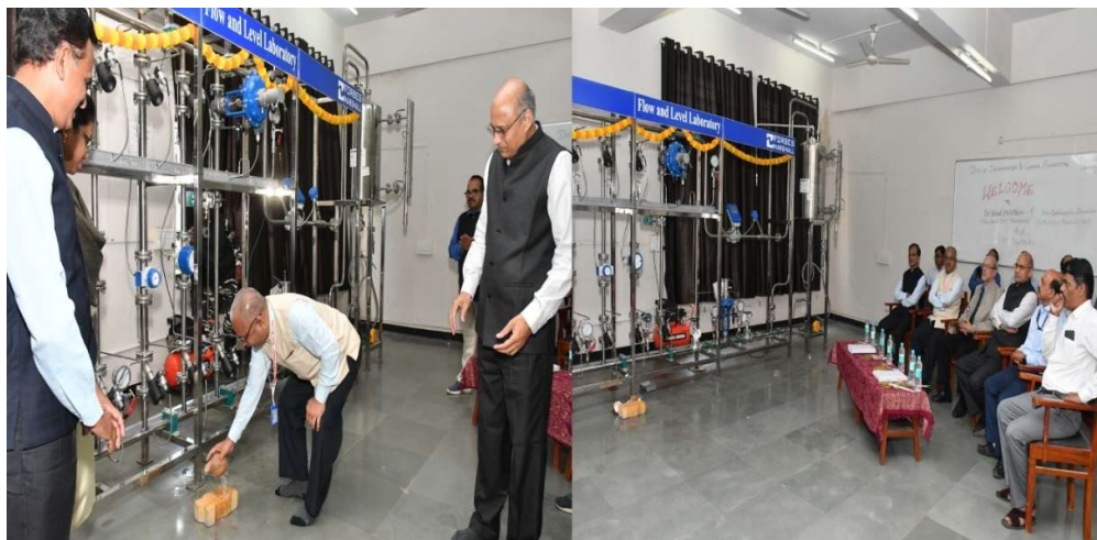
(Flow – Level Laboratory with Modern DCS Setup)
